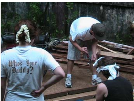
Three 2008 Team Members work on the CMC studio
